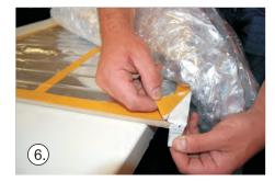
Just peel double sided tape on silver side. Insulation can now be installed on top of heater.
