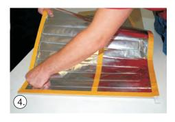
Stick heater firmly down onto board.
