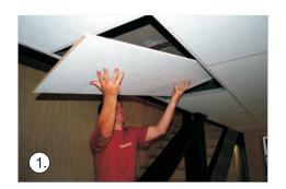
Carefully remove existing ceiling board from ceiling.
