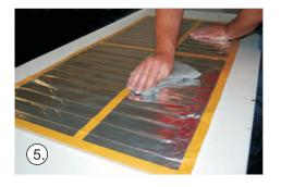
Ensure heater is flush against ceiling board and firmly stuck down into position.
