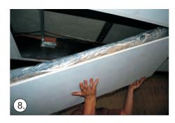
Replace ceiling board with plenty of insulation on top.
