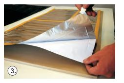
Place heater on top of ceiling board, silver side up.
