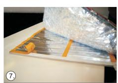
Stick insulation down firmly onto the heater. The double sided tape will ensure heater stays in place.
